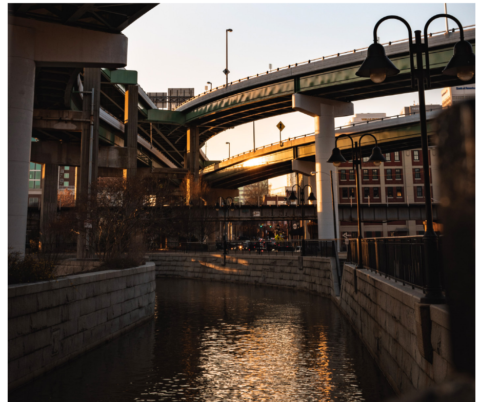
Canal Walk with expressway ramps and elevated rail line (Richmond)
