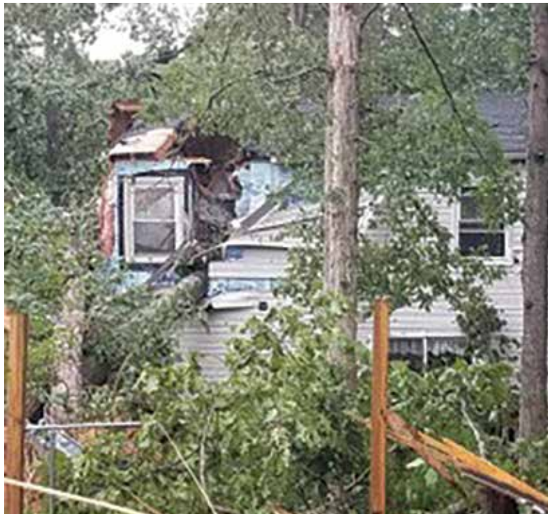
Tornado damage in Chesterfield
