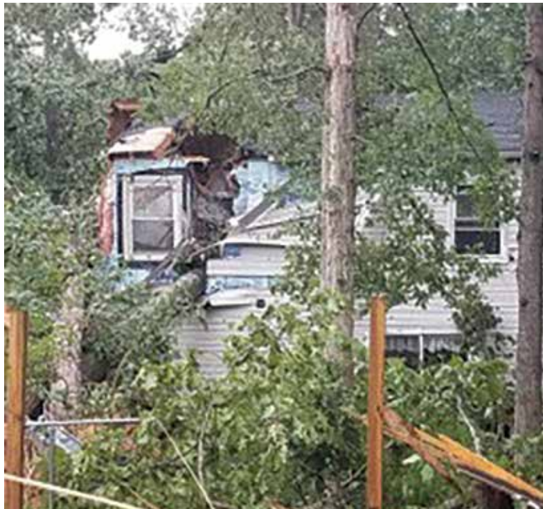
Tornado damage in Chesterfield
