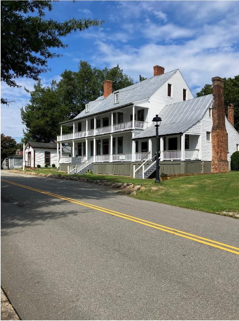
Photo: Atkinson's Hotel, Powhatan Courthouse
