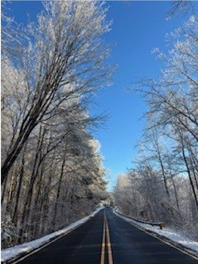
Photo: Sliding Hill Road, Hanover County
