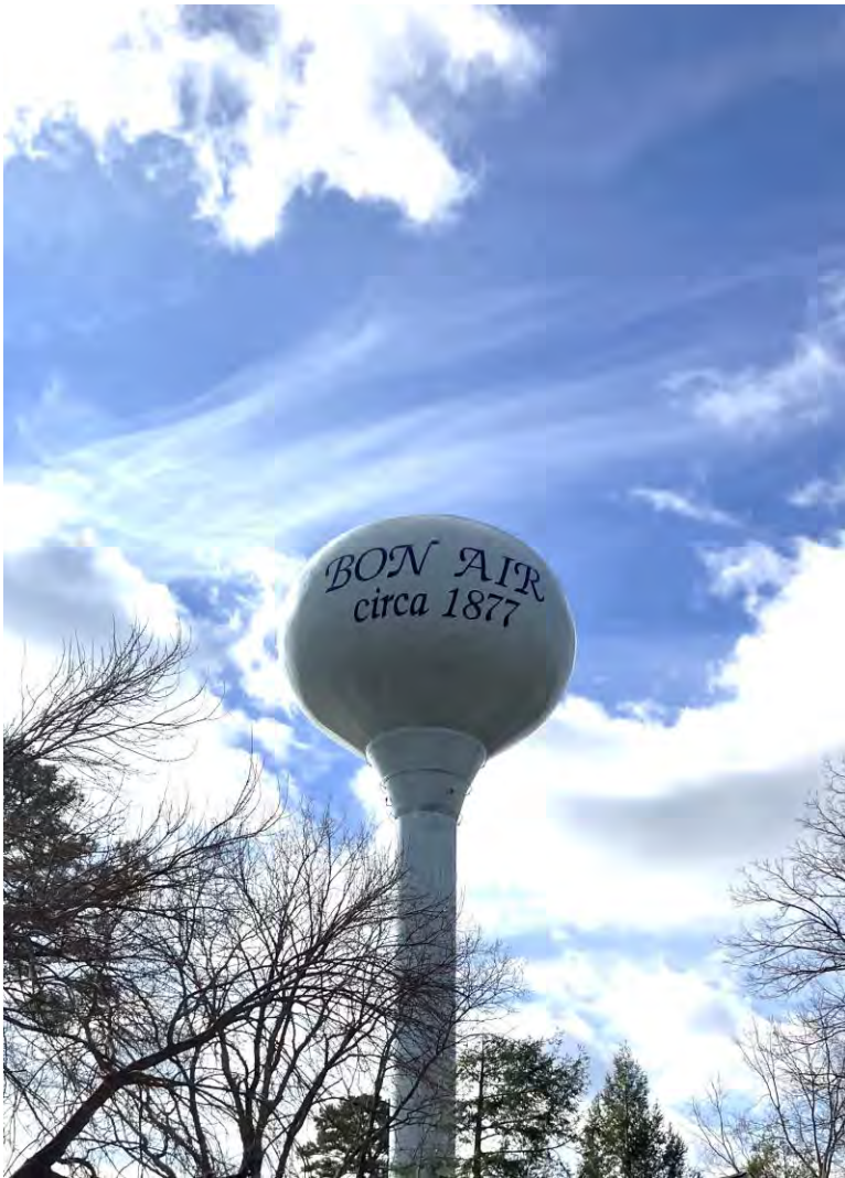
Photo: Bon Air Water Tower, Chesterfield County
