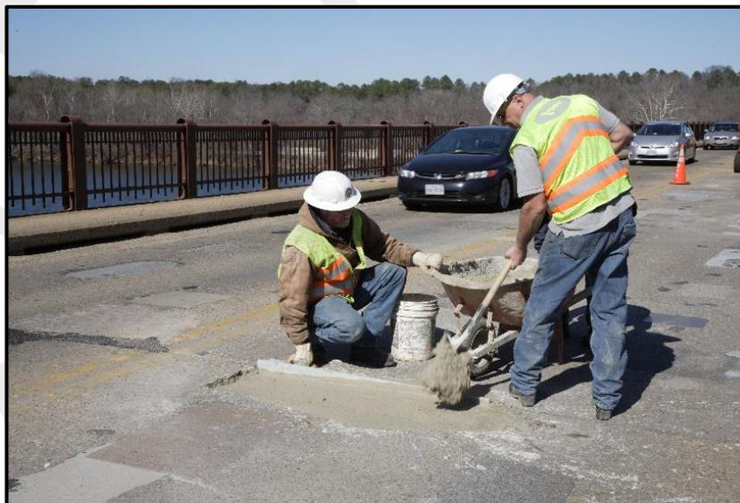
Pouring concrete patches on the Huguenot Bridge (old) deck
