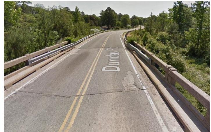
Dundas Rd Bridge deck condition and lack of pedestrian accommodations
