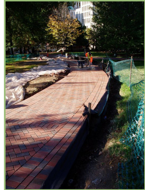
Pervious pavers installed in Capitol Square as part of the Greening Virginia's Capitol project. Source: www.greenvacapitol.org
